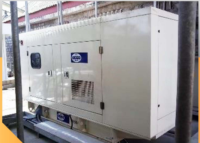
Generator Set Supply, Installation Testing & Commissioning
