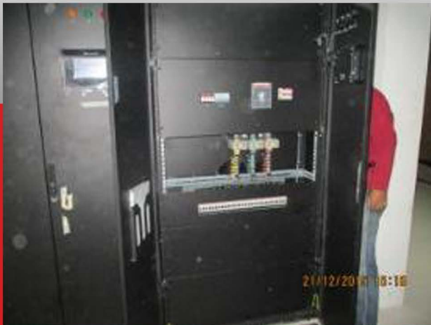
AC PDB Installation
