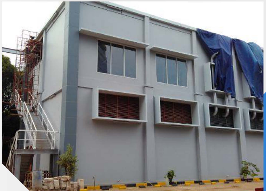
2 Storey Generator Set House 1250 kVA, 6 Unit Designed for Dynamic Load
