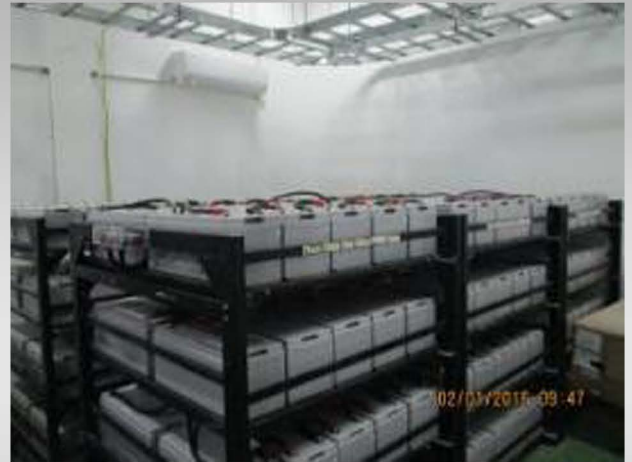
Battery & Racks Installation
