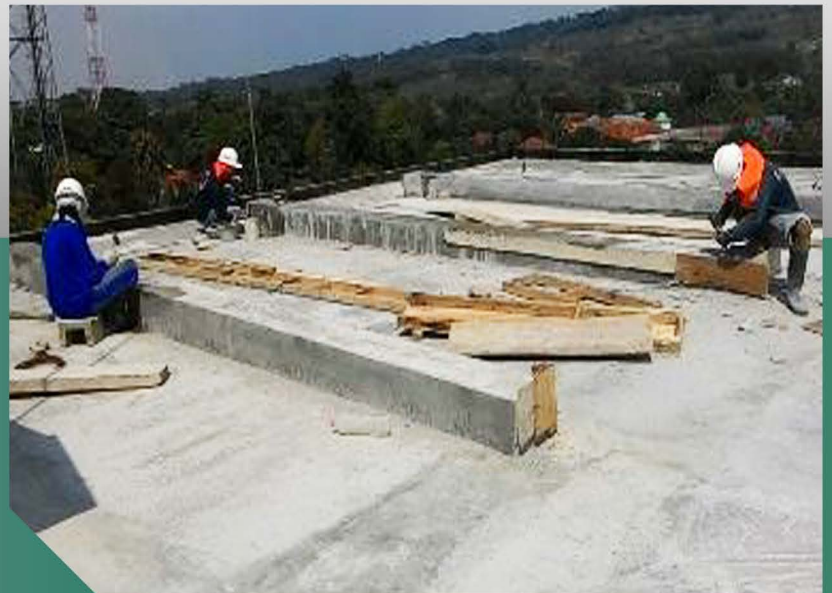
Pouring concrete for Precision Aircon (PAC) Outdoor unit foundation
