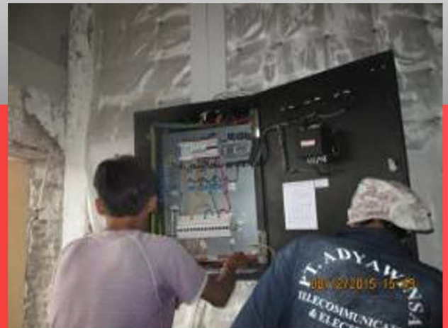
SDP Lighting installation
