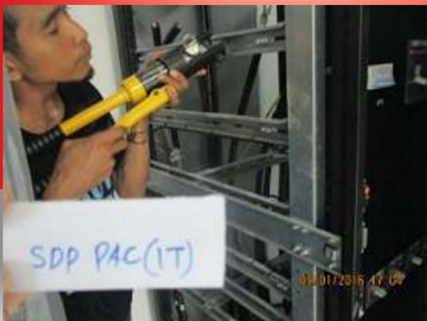
SDP PAC Installation
