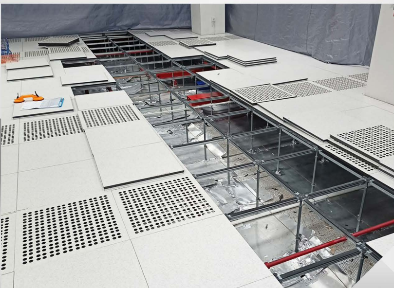
Raised floor work
