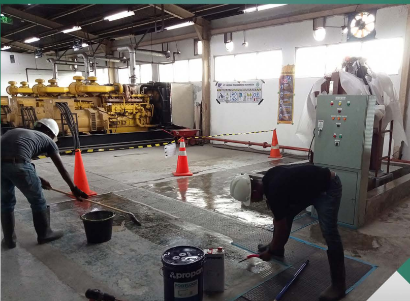
Epoxy Floor Coating
