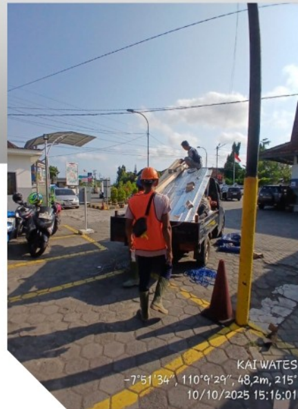
Solar Power Plant Installation Work, Stasiun Wates, Central Java PT KAI (Persero)
