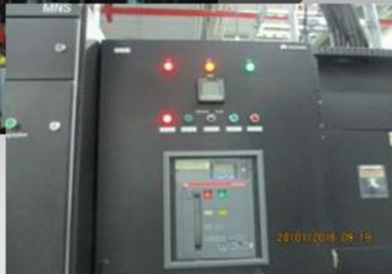
Utility Main Distribution Panel Implementation
