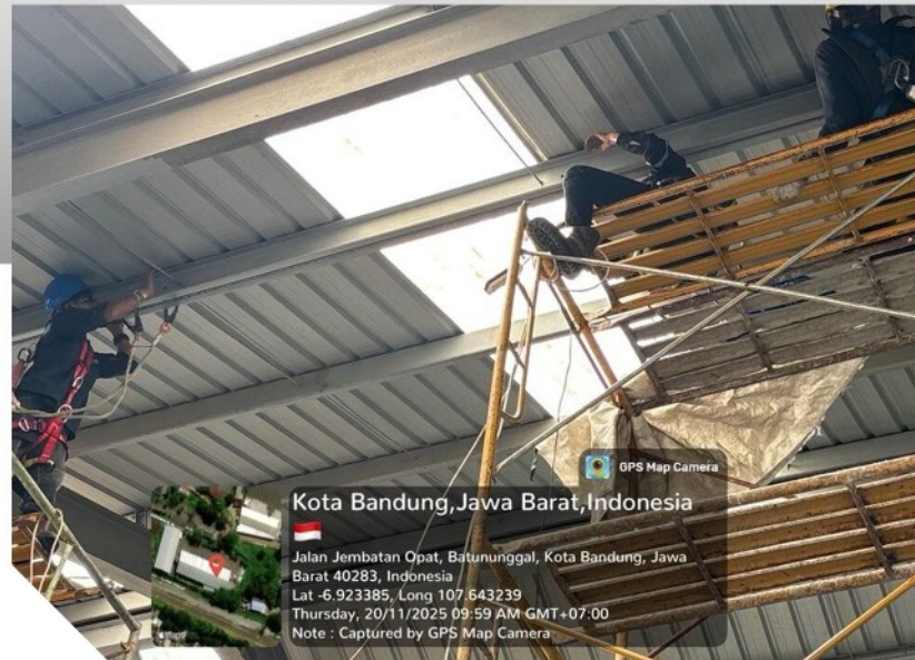
Solar Power Plant Installation Work, Balai Yasa Kiaracondong, West Java PT KAI (Persero)
