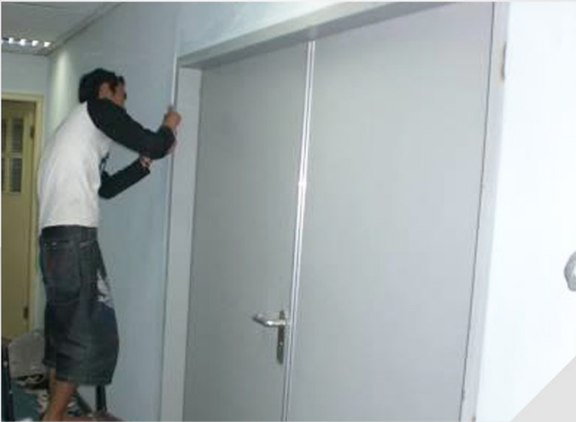
Metal door installation
