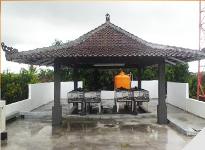
Rooftop : Outdoor PAC, AC Split, CCTV Camera & Bale Bengong as cover outdoor PAC
