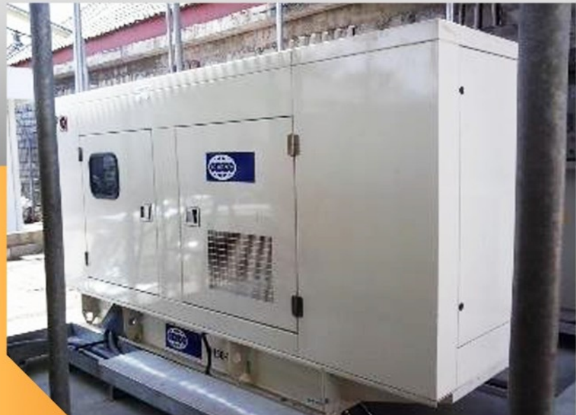
Generator Set Supply, Installation Testing & Commissioning
