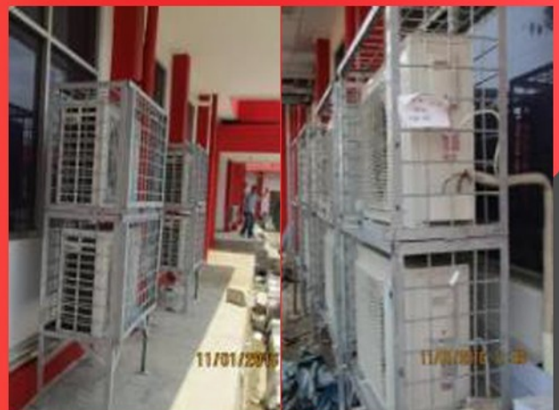
Outdoor Condensor Installation
