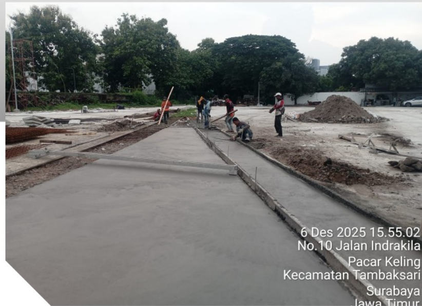
Concrete Road Construction, Street Lighting, and Drainage UPT Gudang Persediaan Gubeng, Surabaya PT KAI (Persero)
