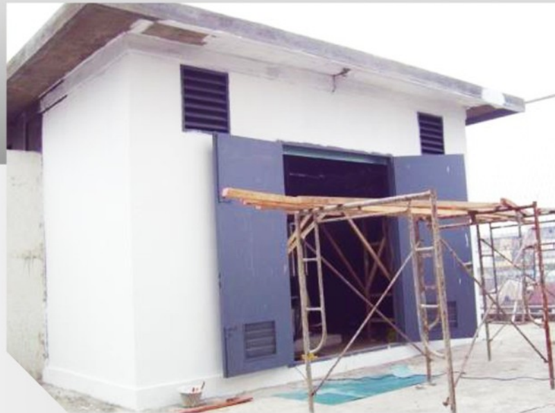
Power / Genset house
