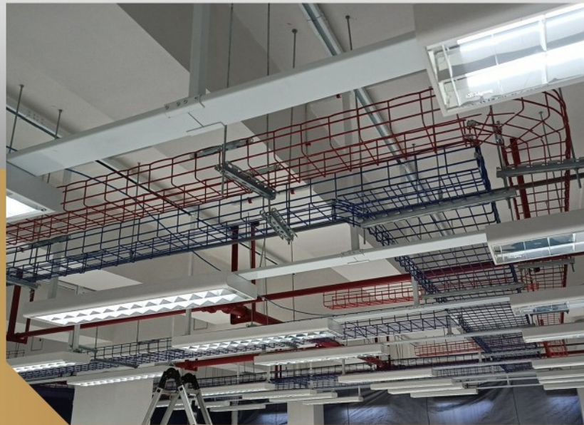
Cable tray installation
