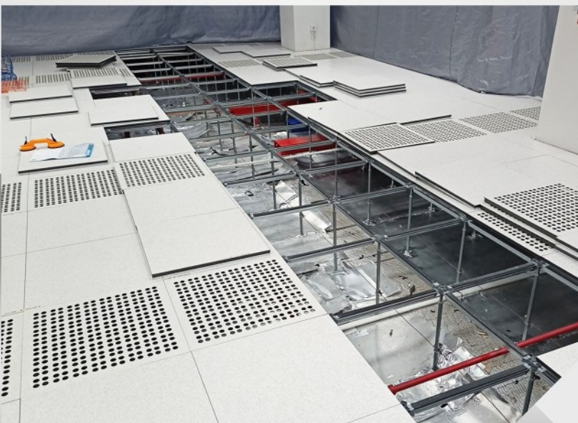
Raised floor work
