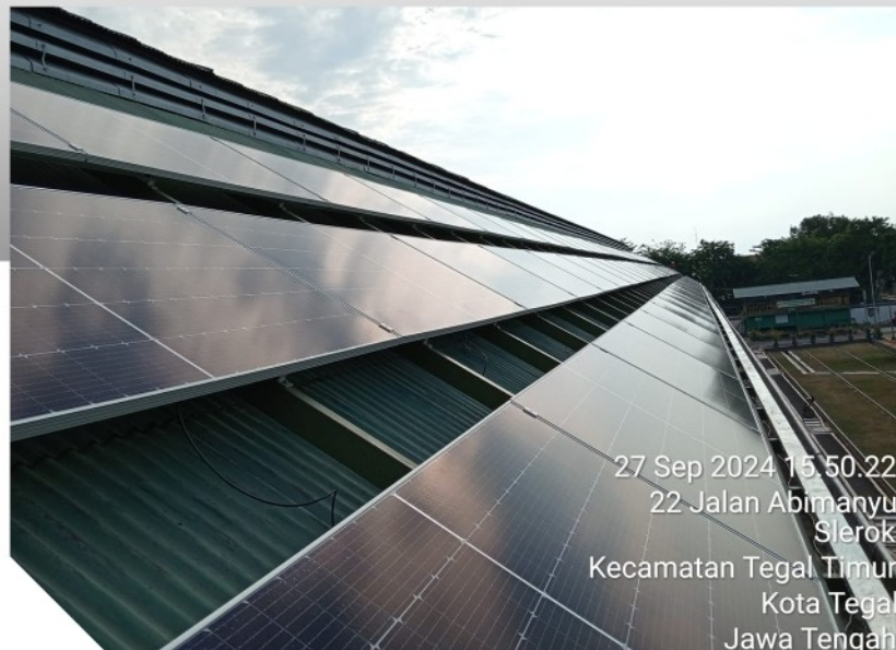
Solar Power Plant Installation Work, Balai Yasa Tegal, Central Java PT KAI (Persero)
