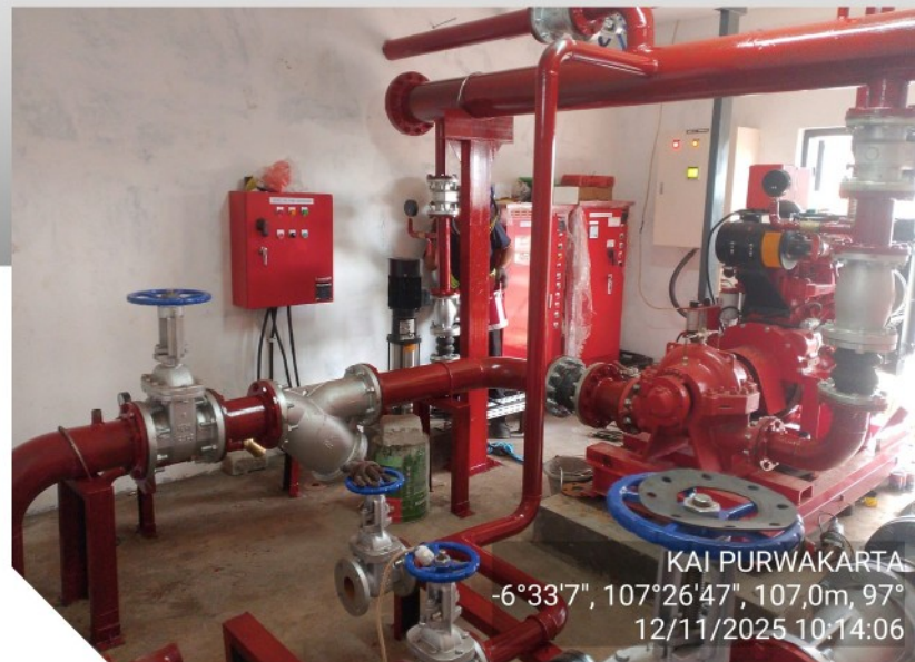
Construction of Pump Houses, Ground Water Tank Fire Hydrants KAI Purwakarta Supply Warehouse PT KAI (Persero)
