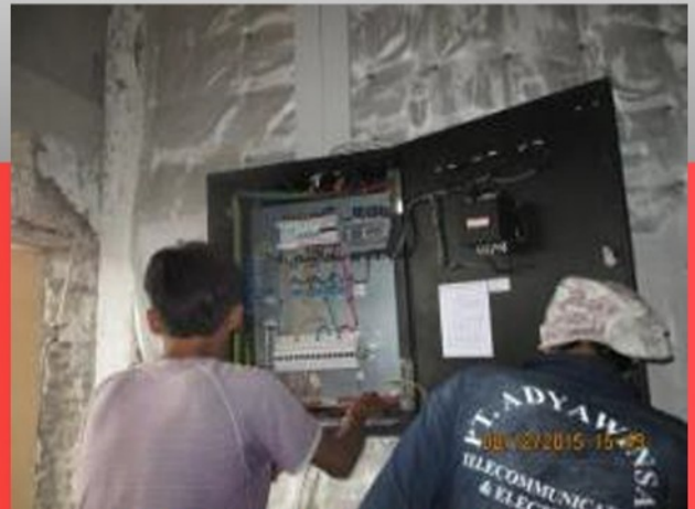
SDP Lighting installation
