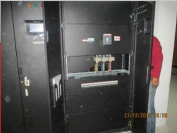
AC PDB Installation
